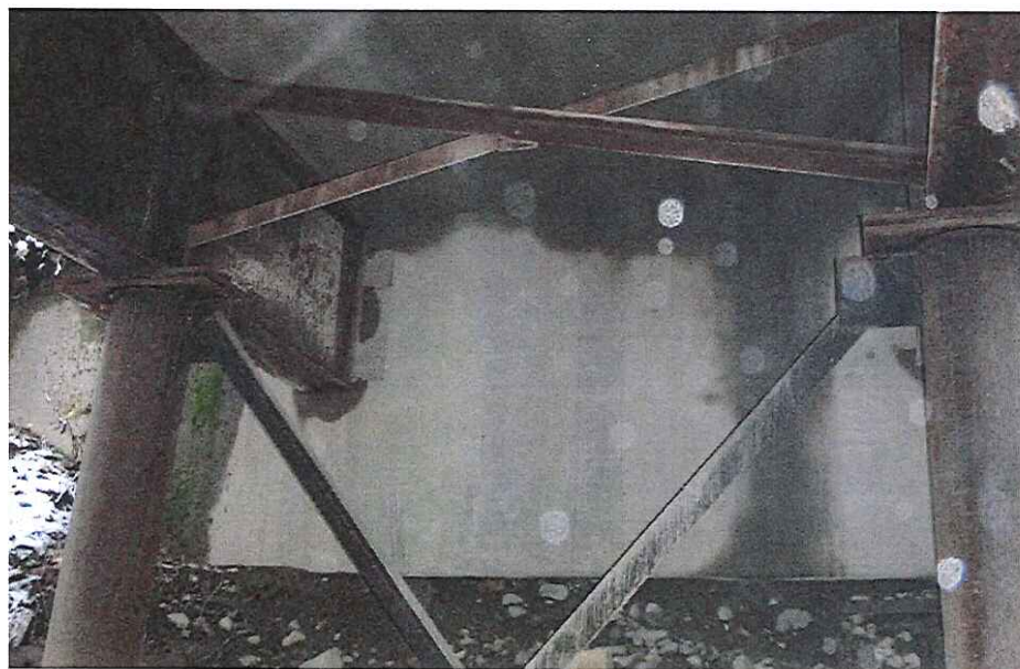
CK-2047 Abutment Right Bank
