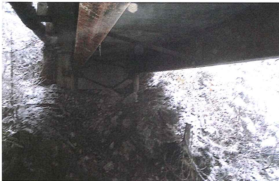
CK-2047 Abutment Left Bank
